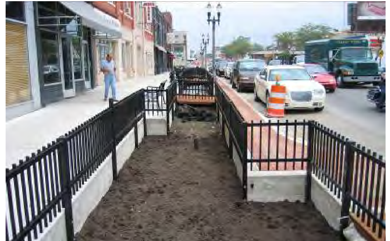
Main Street during construction
