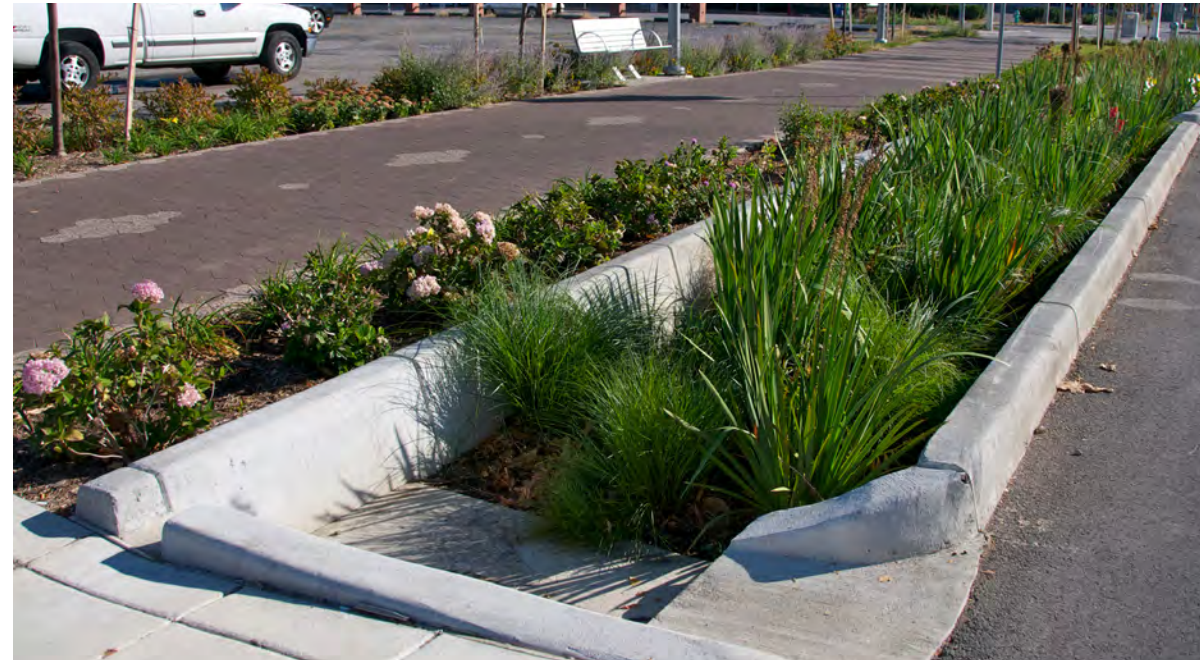
A bio-retention swale and the Trail between parking lots and the street.
