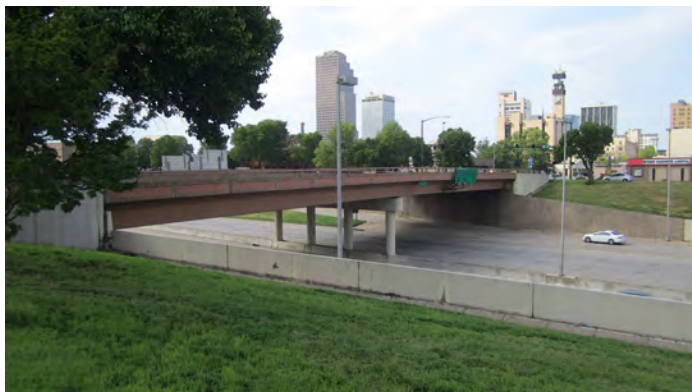
EXISTING VIEW (Bridge over highway 630, from southeast)
