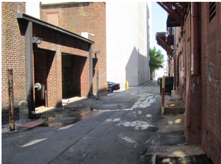
EXISTING VIEW (Alley east of Main between 6th and 7th)
