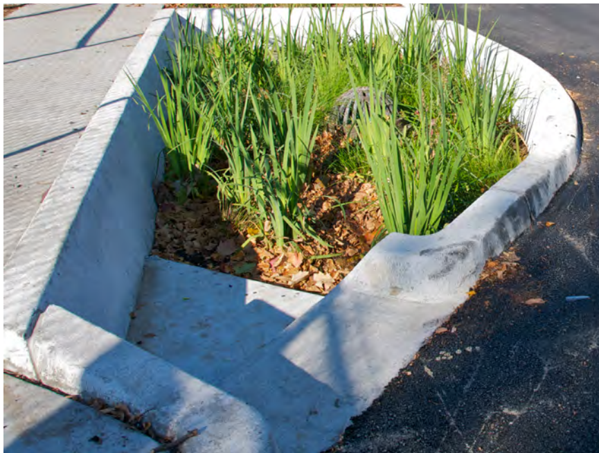
A corner bio-retention basin.
