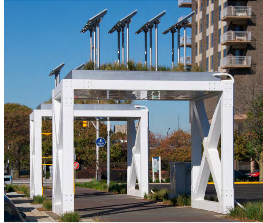
"Prairie Modules 1 & 2" references our agricultural and urban environment and is designed to invite spatial interaction and experiential awareness. Through a partnership with Indianapolis Power & Light, this is the first public art installation in Indianapolis to return solar power to the electrical grid.
