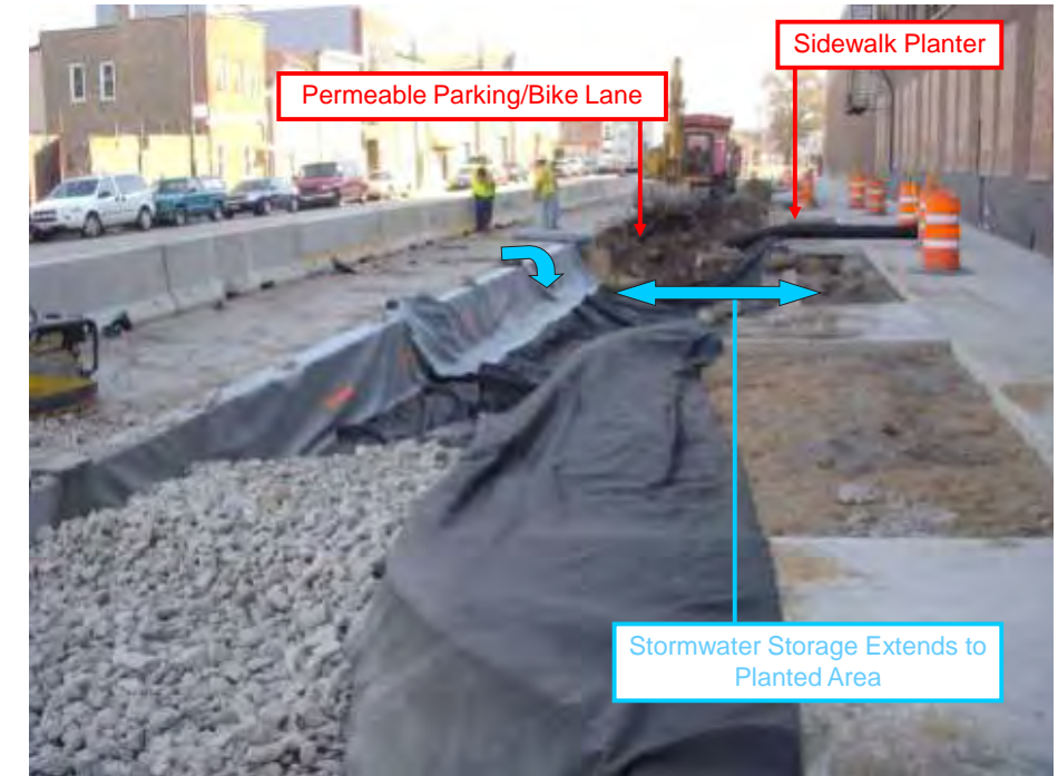
Cermak Road during and after construction of permeable parking, stormwater storage, and sidewalk planters.
