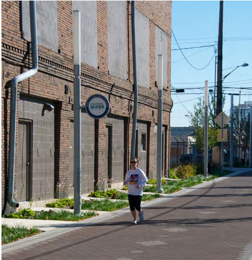
Downspouts flow into stormwater basins along the Cultural Trail.
